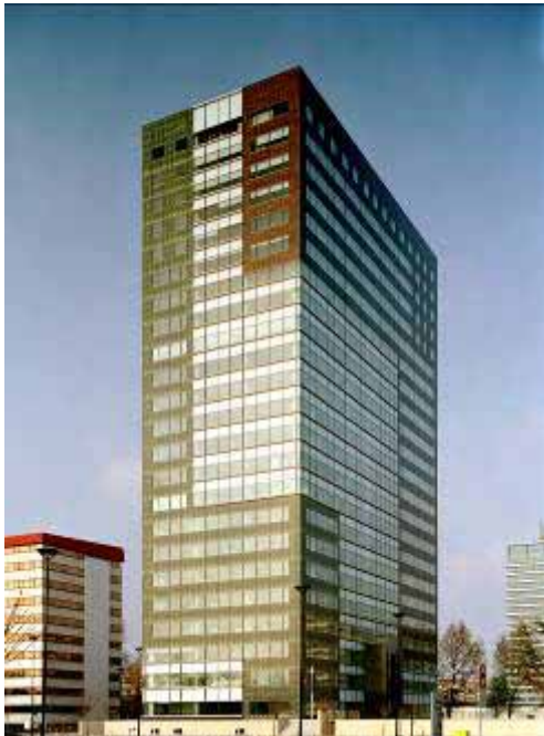
Winston Churchill Tower - Rijswijk: Renovation with a double skin facade (internally ventilated) Source: Permasteelisa Group
