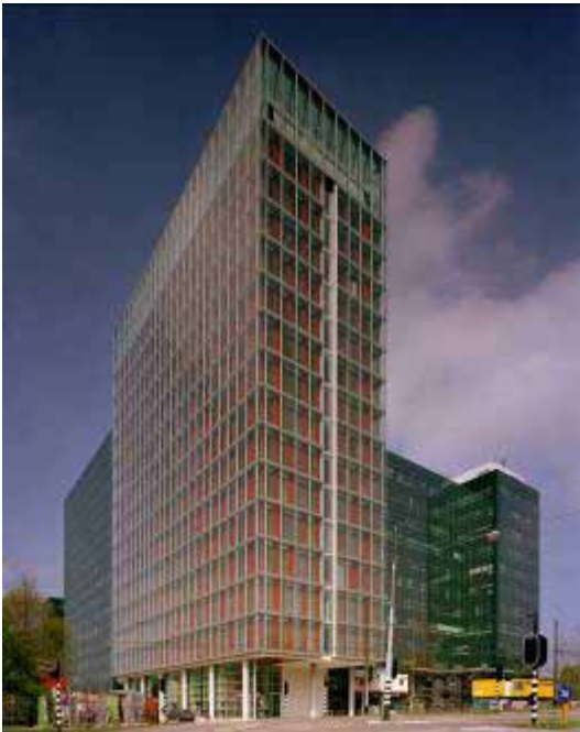
World Trade Center - Amsterdam (WTC): Renovation + extension of an office building Source: Permasteelisa Group
